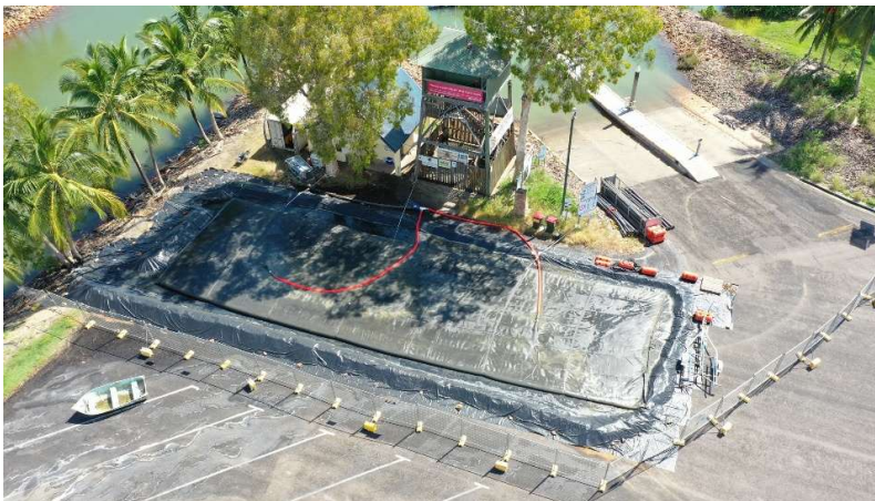
Boat ramp area
